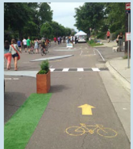
Tactical installations can increase access for pedestrians through bike lanes, landscaping, and parallel parking. These narrow the street and reduce speeding, making the right-of-way safer for pedestrians
