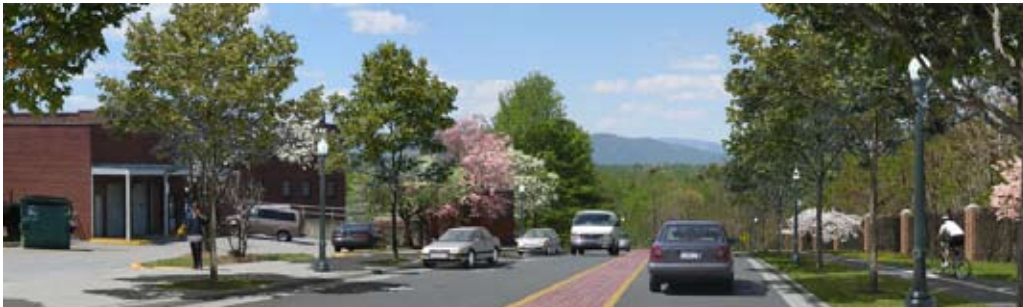
Short-term Improvements: Lakeside Drive is widened to accommodate on-street parking. A brick safety zone in the middle would be utilized by ambulances making their way to Lynchburg General Hospital. Street trees and a new sidewalk are added. A new fence is constructed along the E.C. Glass High School property.
