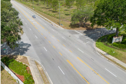
Burns Avenue and Tower Road redesign
