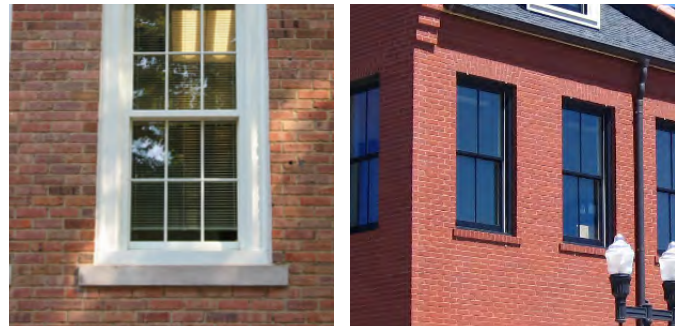
Figure 405.14.E.2.b Sills. Cast Concrete (left) and Brick (right)
