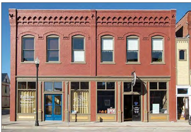
Figure 405.12.G: Examples of Live/Work Buildings:
