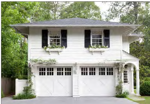
Figure 405.12.Q: Examples of Carriage House Buildings:
