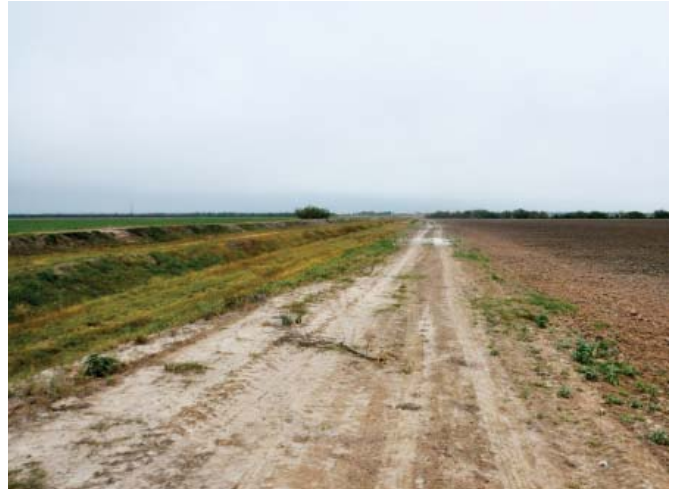
Existing dirt roads along irrigation canals for existing farm fields.
