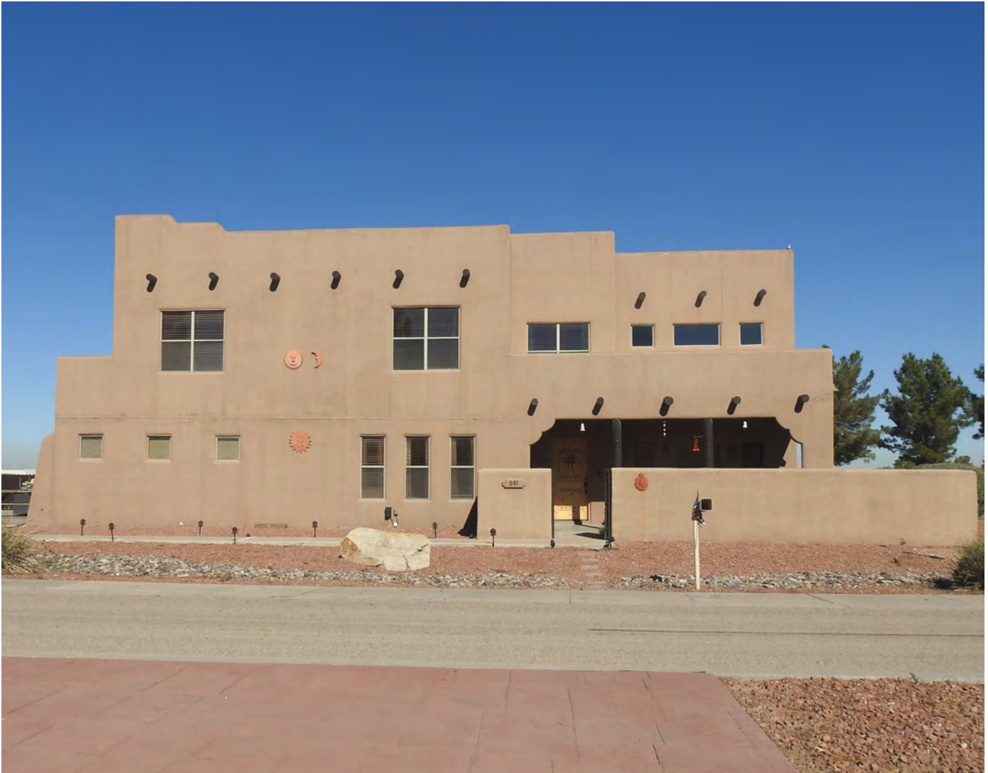
Apartments with Pueblo Style Architecture
