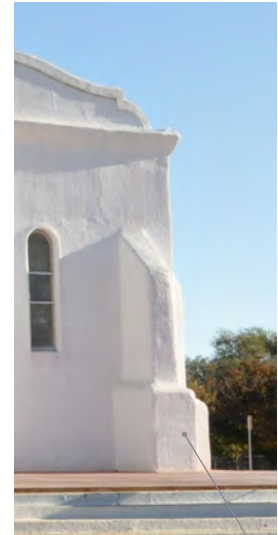
buttresses and wing walls
