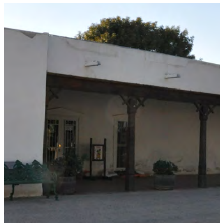
Typical roof in the San Elizario Historic District with scuppers, parapet roofing and wooden porch
