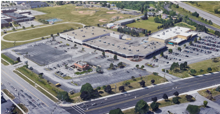
BELOW: Existing Conditions, Boulevard Mall
