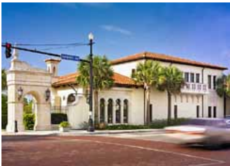
The new Marshall and Vera Lea Rinker Building was designed to engage the McKean Gateway on the southwest corner of Park and Fairbanks Avenues.
