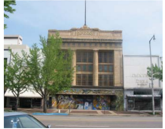
Many façades along Dexter Avenue are in need of repair.
