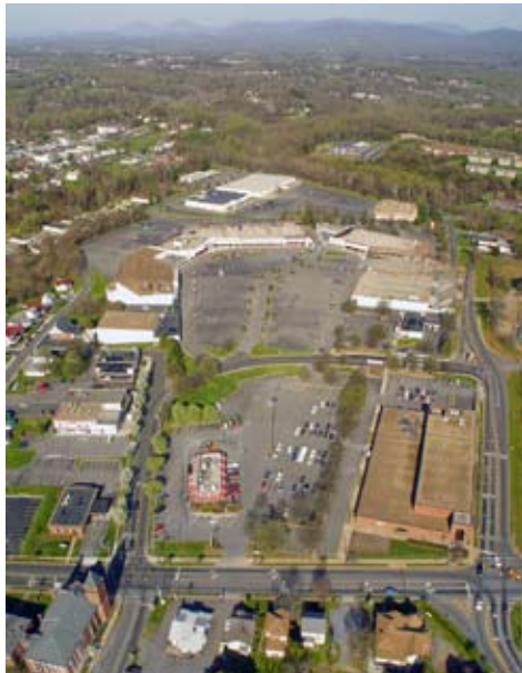
Above: Existing aerial view of the Plaza.
