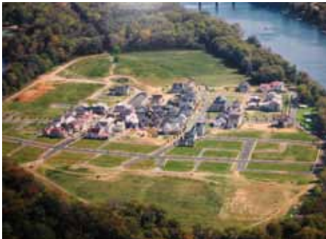
Phase One development of Hammond's Ferry is underway, with the first homes constructed in the heart of the neighborhood.
