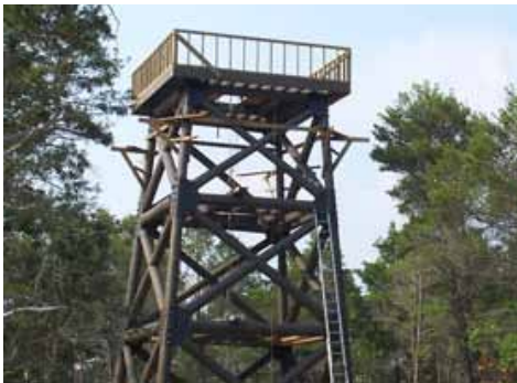
A 48-foot observation tower, built of heavy timber and steel, is an architectural centerpiece of Draper Lake, providing panoramic views of the neighborhood and Gulf of Mexico from within the central neighborhood green.
