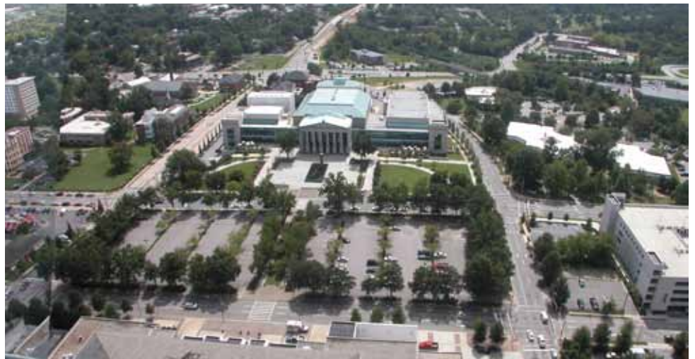
Existing conditions of the BTI Center and public open space at the southern terminus of Fayetteville Street.
