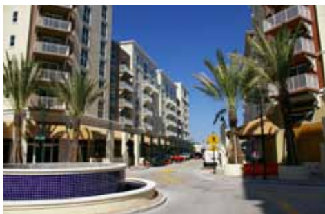
Shops and restaurants occupy the ground floor along the main street.
