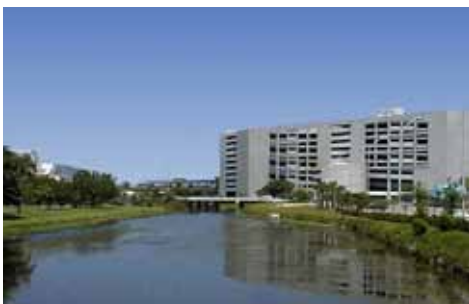
Snapper Creek Canal: Before
